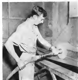
Prop blade gets working over in being polishing department designed and built during war by Southwest Aircraft's master technicians. This shop is maintained in accordance with Hamilton Standard specifications. (Tom Collier photo)
